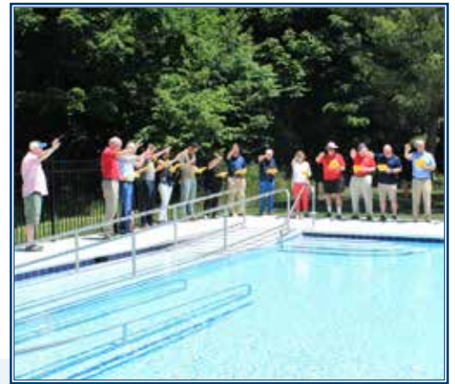
The renovation of the pool was a major accomplishment. The project was completed in time for our campers to enjoy this summer. Above, staff and board members gather for a blessing before the beginning of the camp season.
